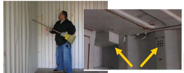
**i** Any repairs on the inside must be also visible on the outside. Blocks and vents (9 holes) inside container must be visible and appropriately spaced (see above picture).
