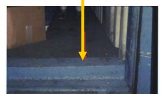
**i** You should not need to step up from edge of container to get inside; there should be no steps or raised platforms inside container.
